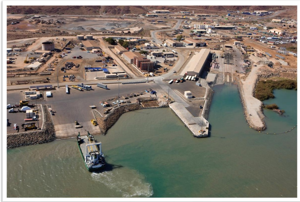
Figure 10 – Supply Base RoRo and Slipway Access
