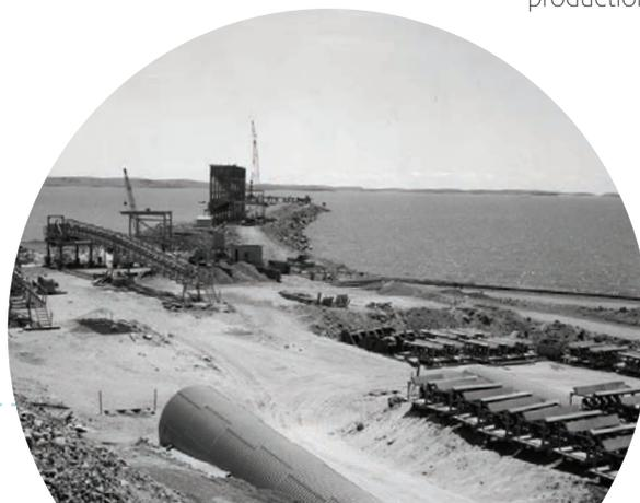
Construction of iron ore processing plant and export facilities at King Bay (Dampier), 1966.
