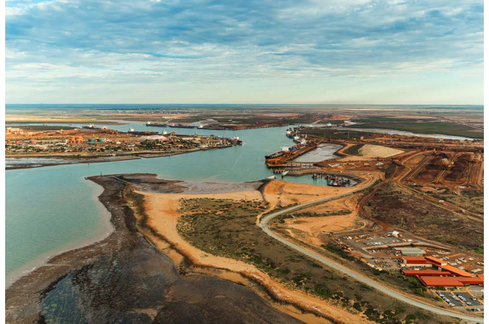
Port of Port Hedland
