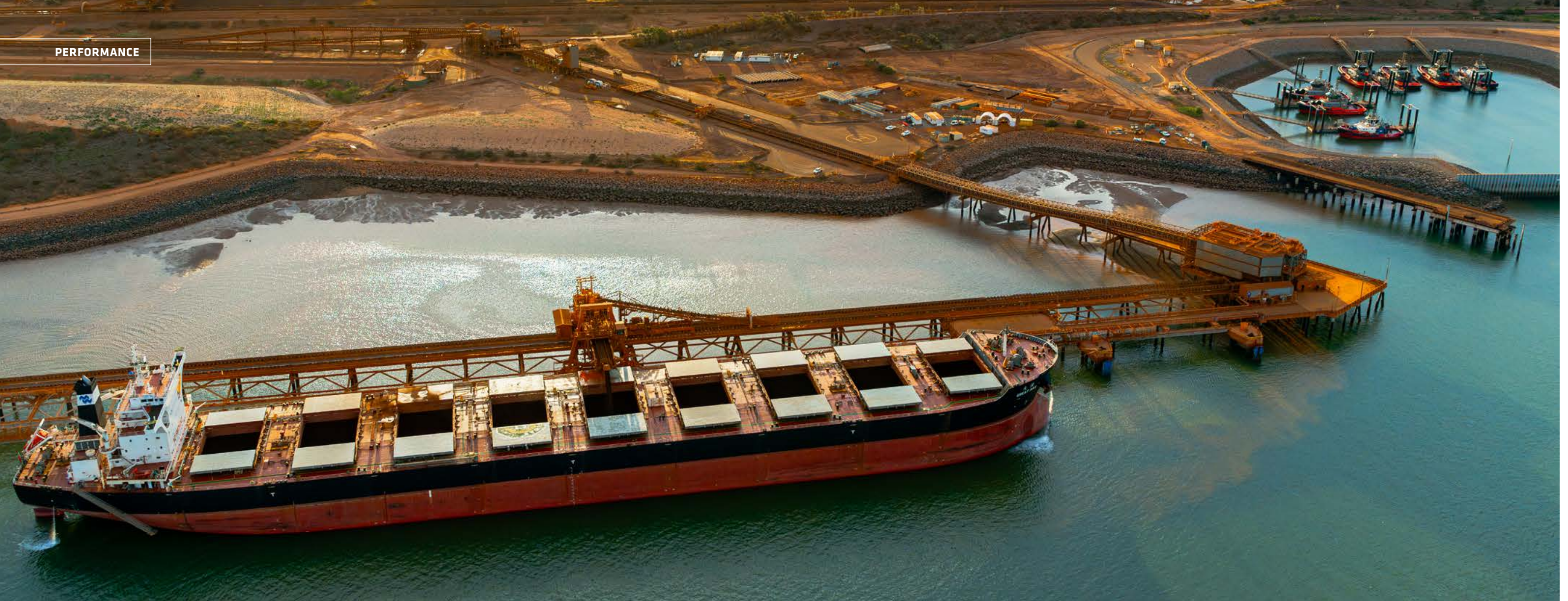
Port of Port Hedland
