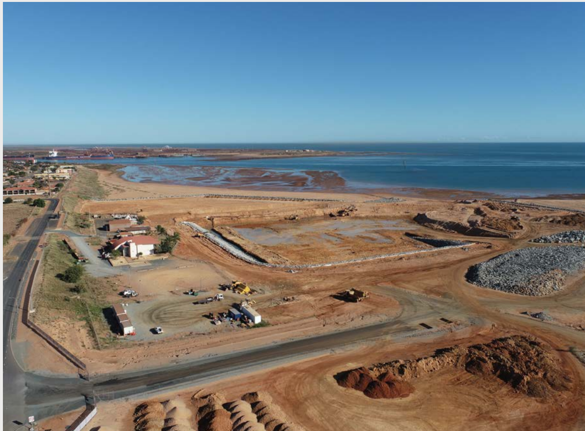
The Spoilbank Marina work site in June 2022.
