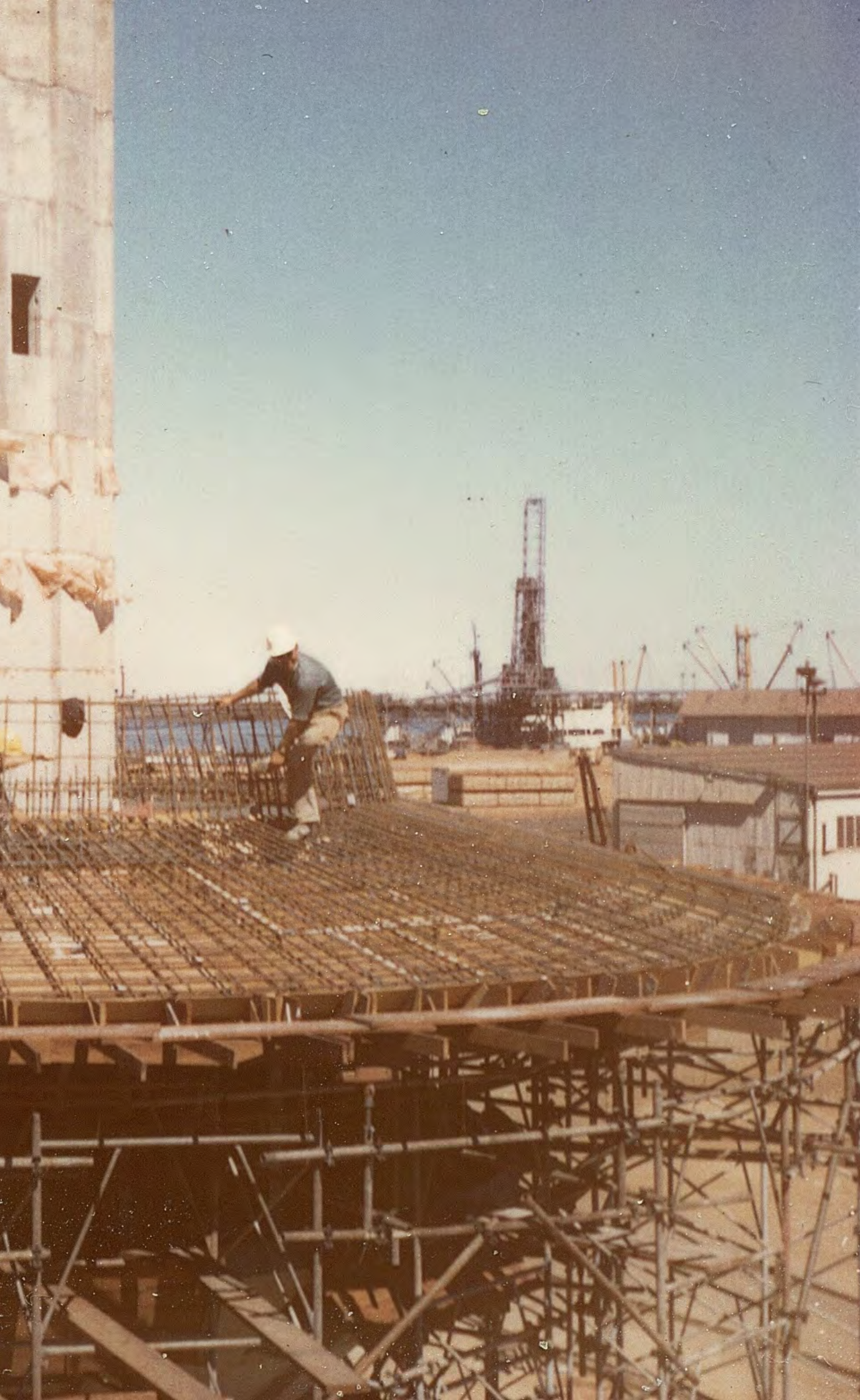
Reinforced steel of the observation element, 1969
