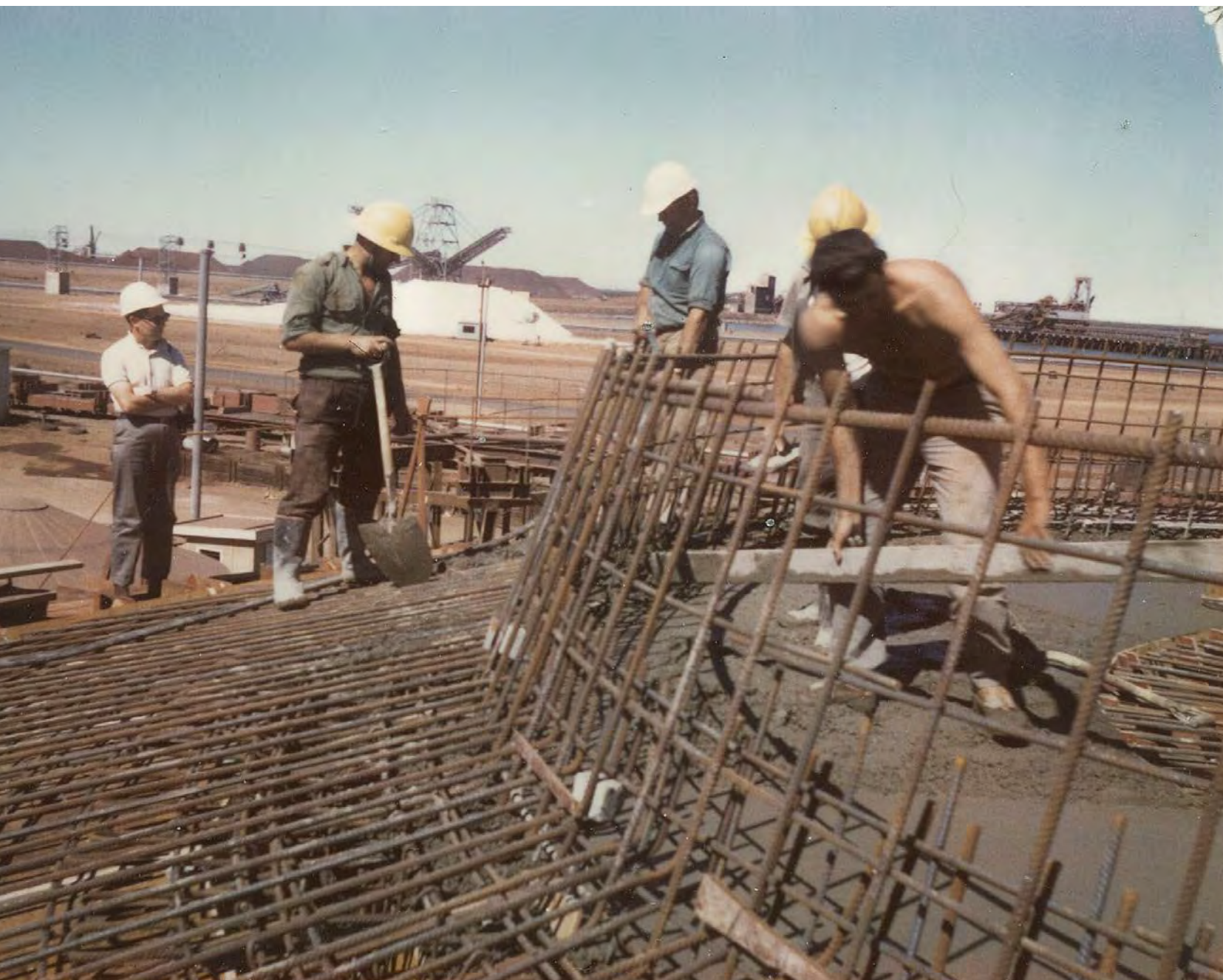
Concreting over the reinforced steel of the observation element, 1969
