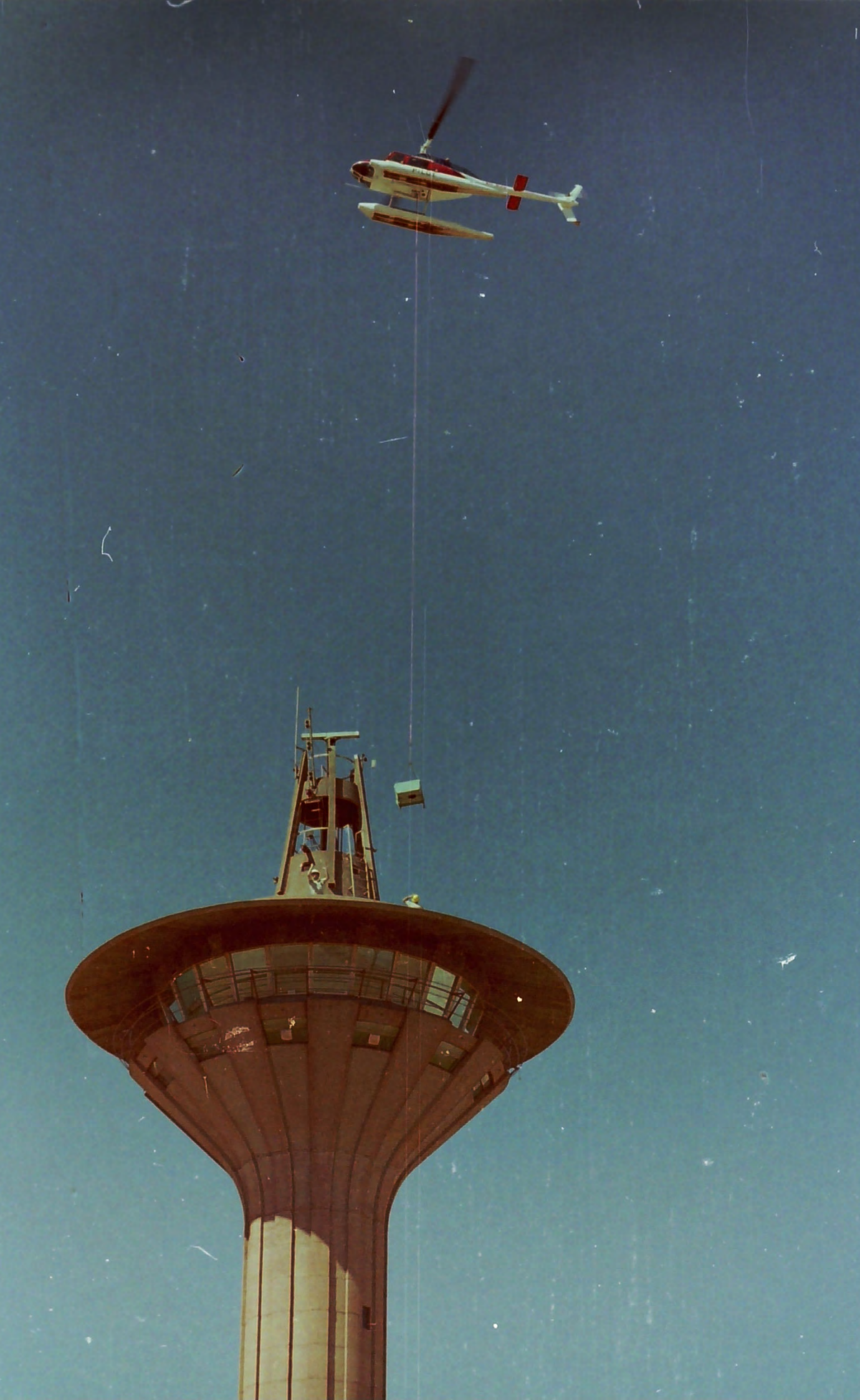
Equipment being helicoptered onto the top of the tower
