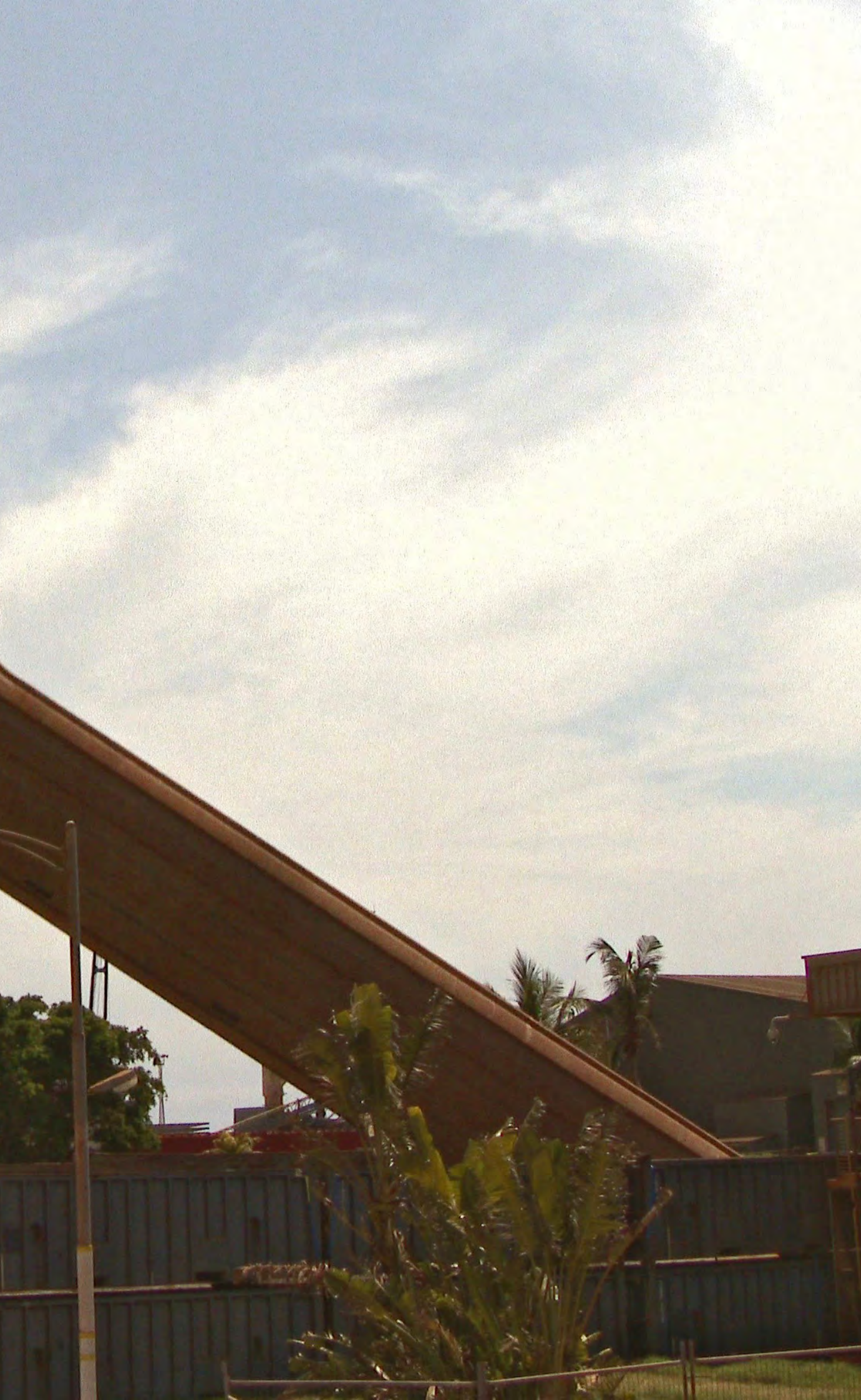
Heavy equipment pulled down the tower using ropes fixed to the upper levels.
