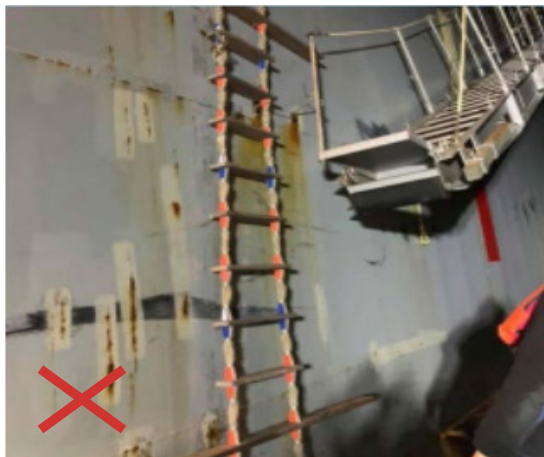
Distance of combination ladder from water line less than 5 metres
