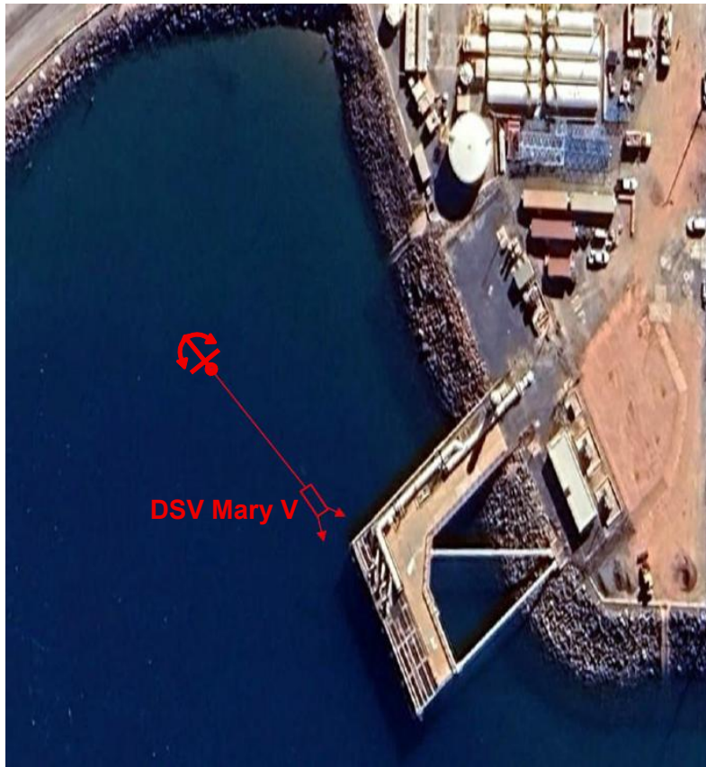
DSV Mary V - Stern anchor location (North): 20° 37.839'S // 116° 45.084'E
