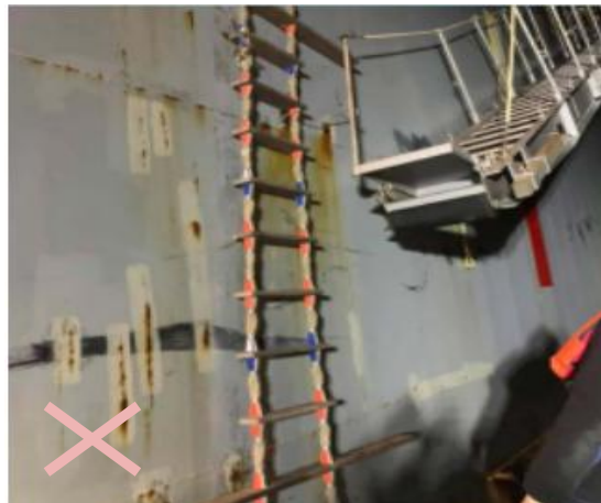
Non-compliant combination ladder arrangement
