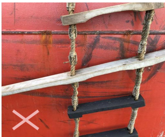
Loose ladder steps & not horizontal
